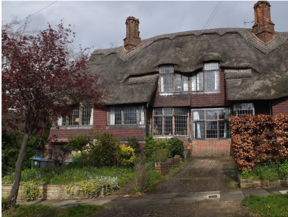
Ernest Trobridge, Buck Lane, Kingsbury, London, ca. 1920s.
